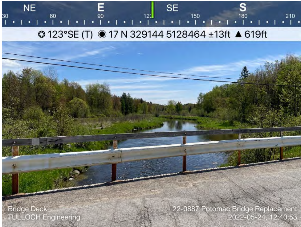
Photo 3: View from bridge deck facing southeast
