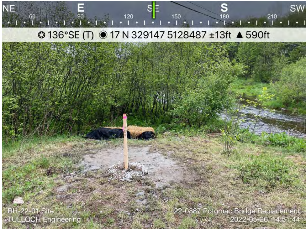
Photo 7: BH-22-01 location borehole backfilled
