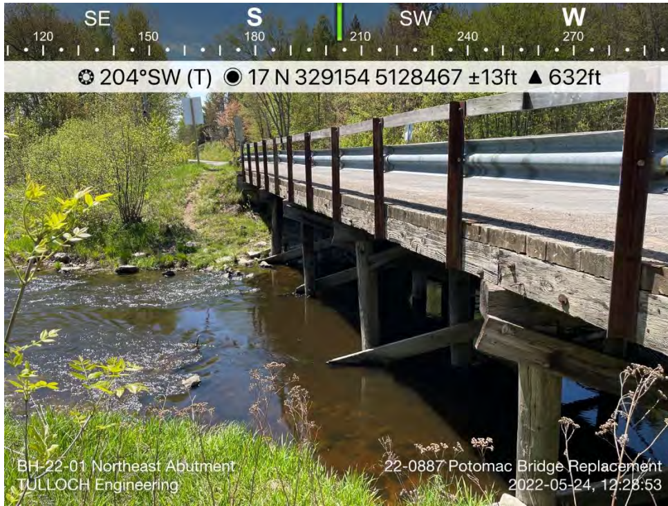
Photo 5: View of existing bridge deck and foundation from north abutment
