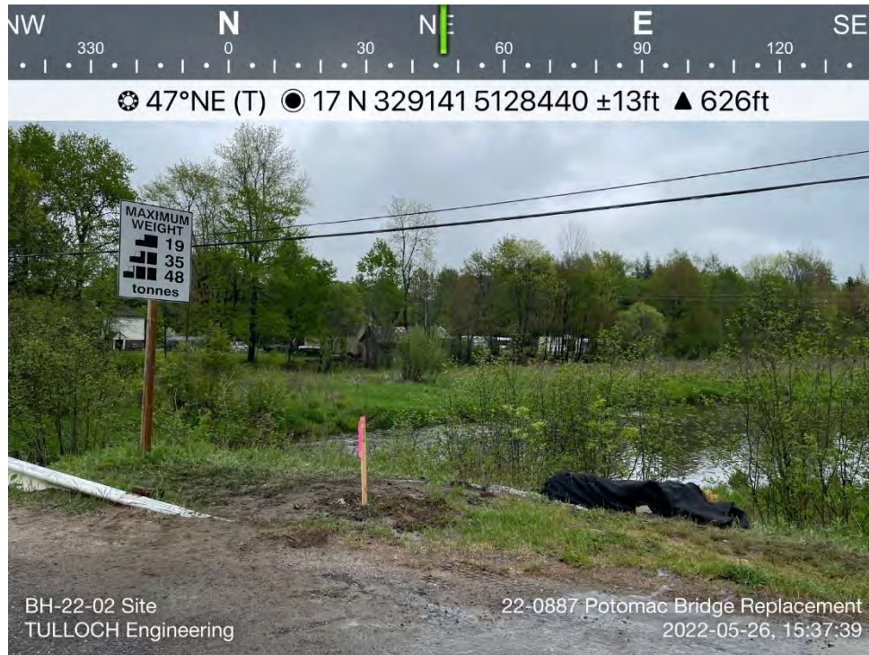
Photo 8: Completed BH-22-02 and backfilled
