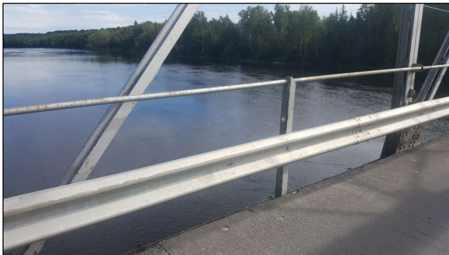
Figure 7 - Typical Guiderail and Railing on Structure
