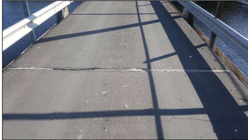
Figure 6 - Typical Deck Joint
