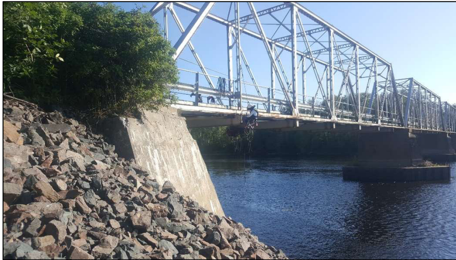
Figure 18 - Rock Protection in NW Quadrant Only
