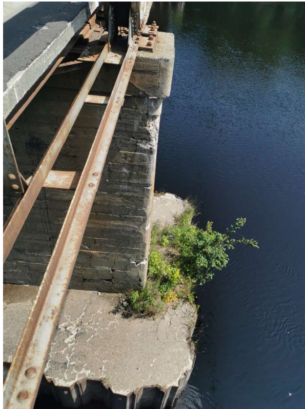
Typical Bottom Chord - Double angles
