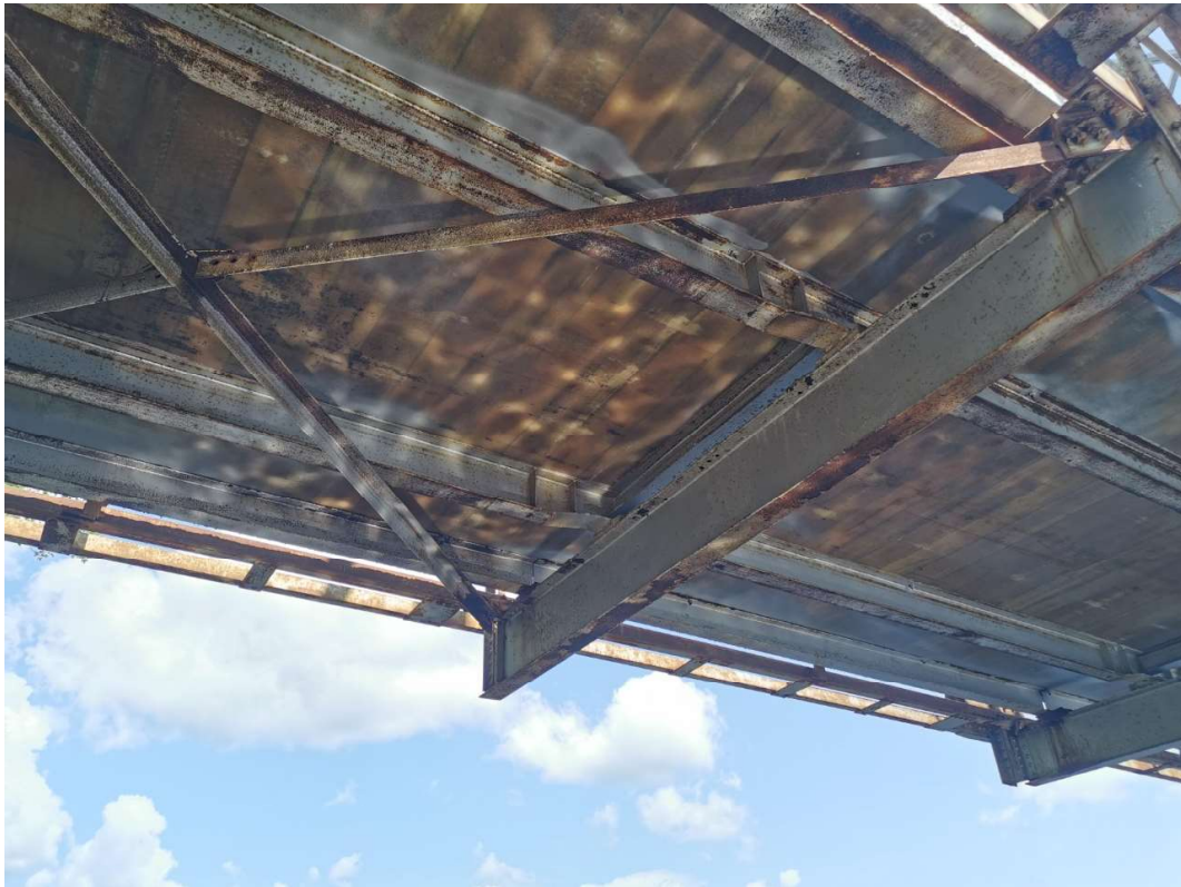
Steel Stringers within Middle Sections
