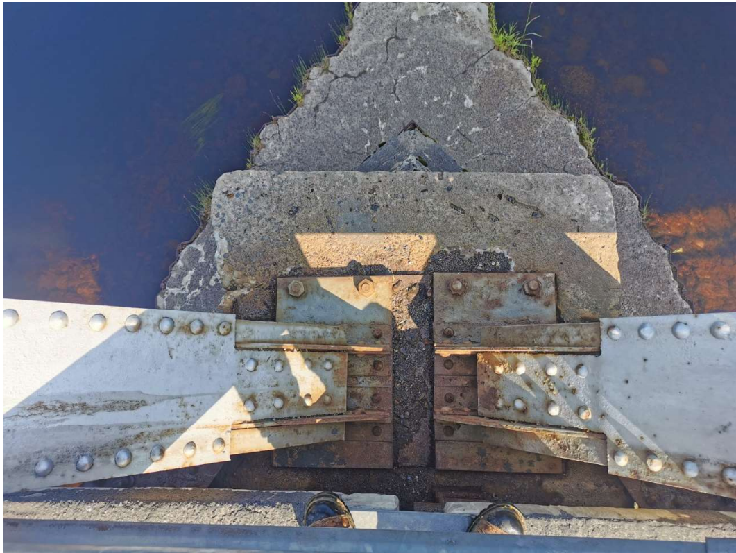
Typical Pier Bearing (North Pier)
