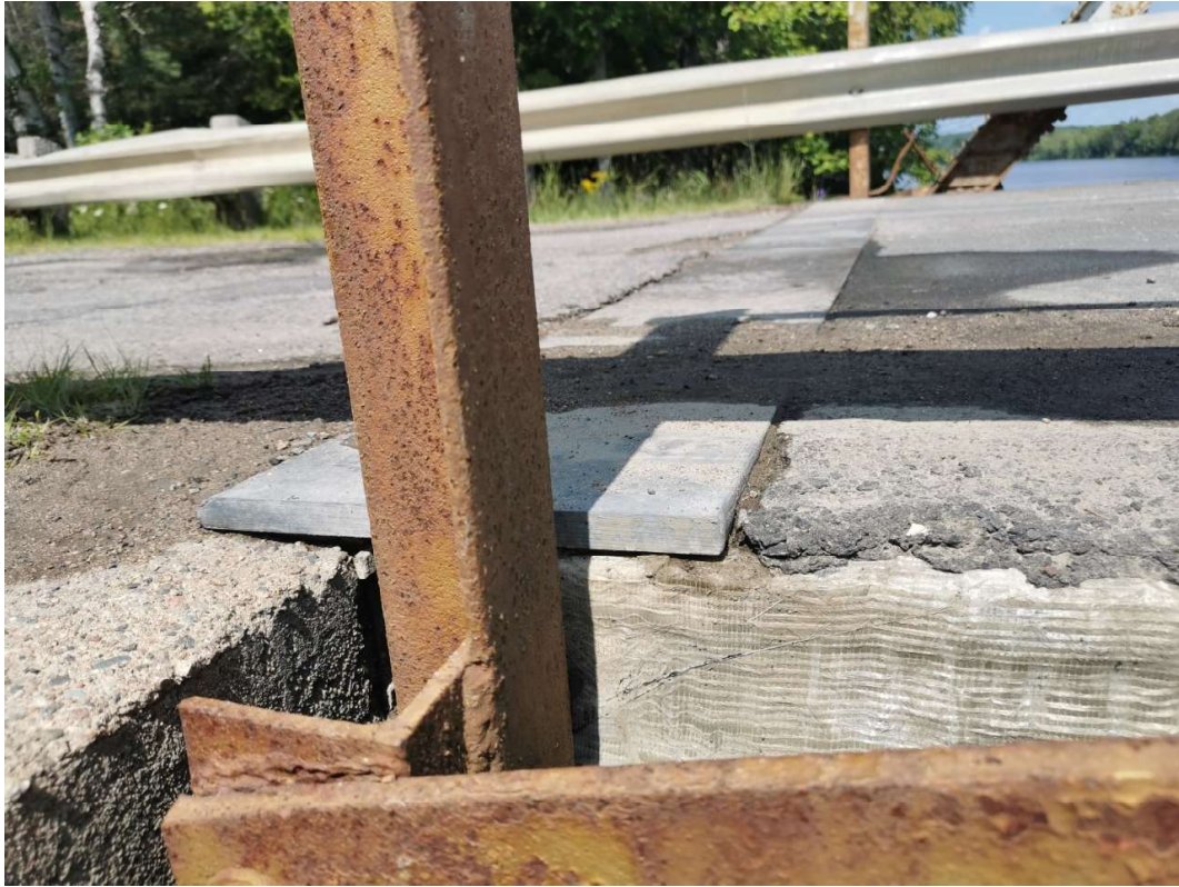
Typical Concrete End Dam
