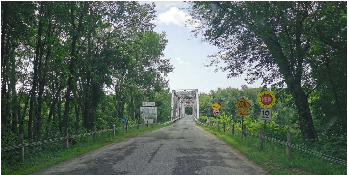
Looking South Across Structure
