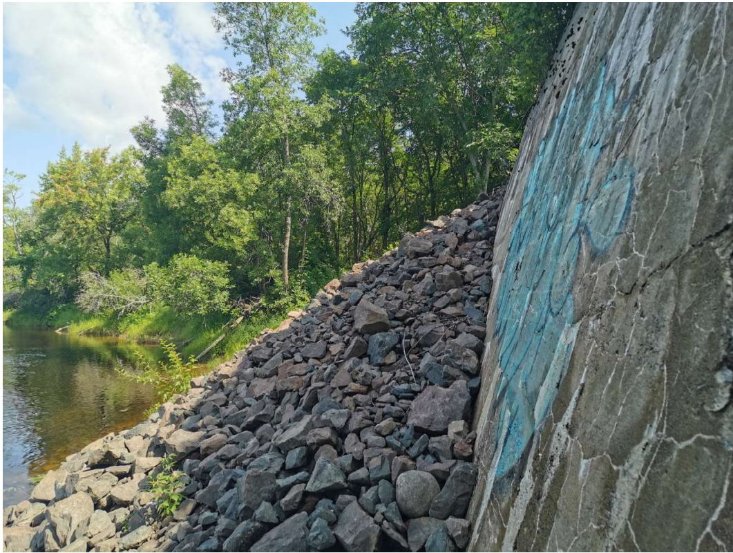
Rock Protection on NW Embankment
