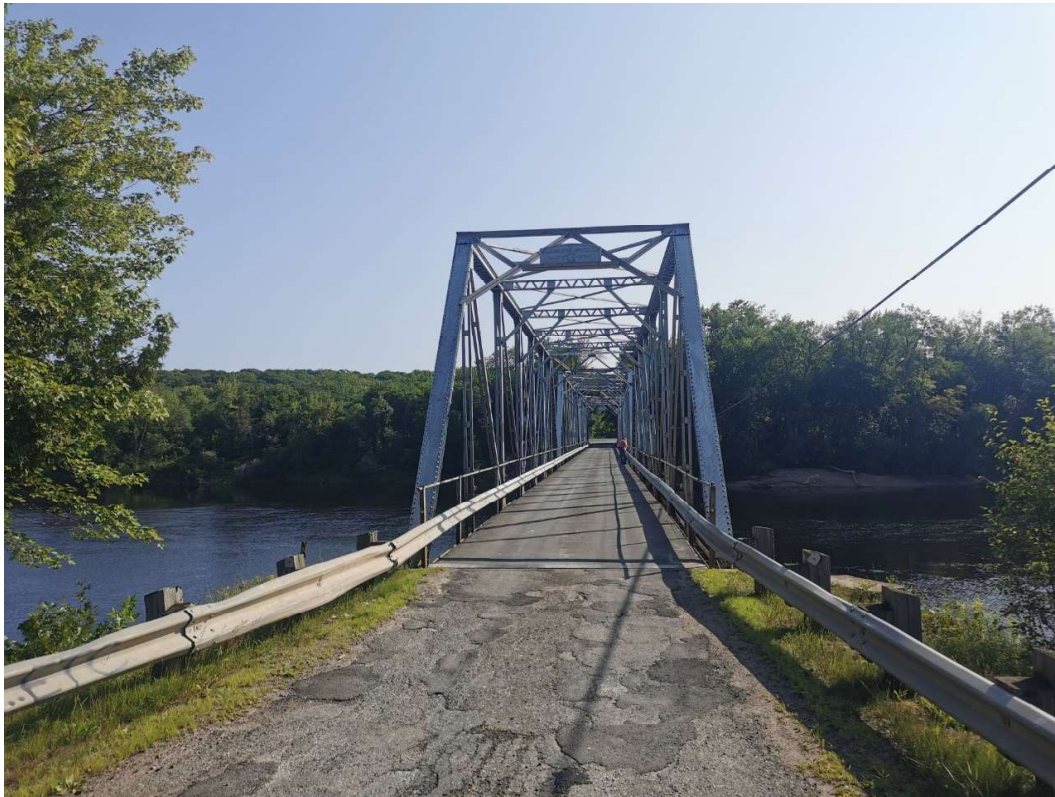
Wooden Posts with Moderate to Severe End Decay.
