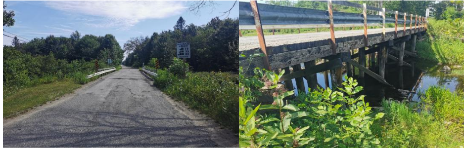
Looking South Across Structure
