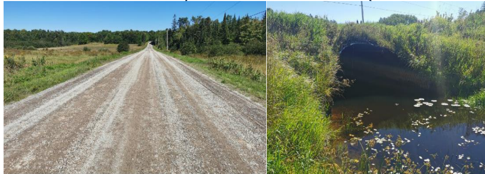
Looking North Across The Structure
