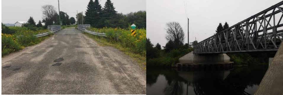
Looking East Across The Structure
