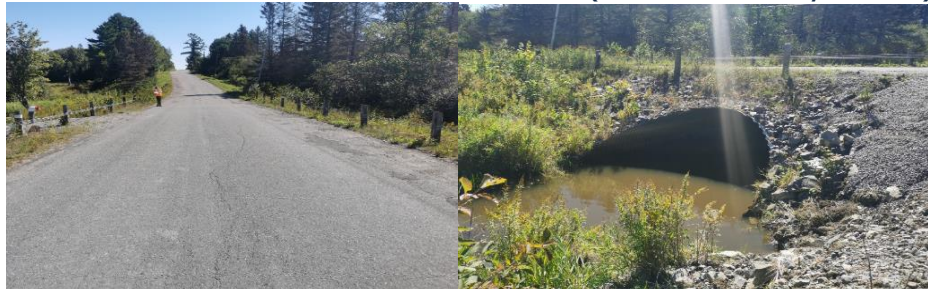
Looking East Across The Structure
