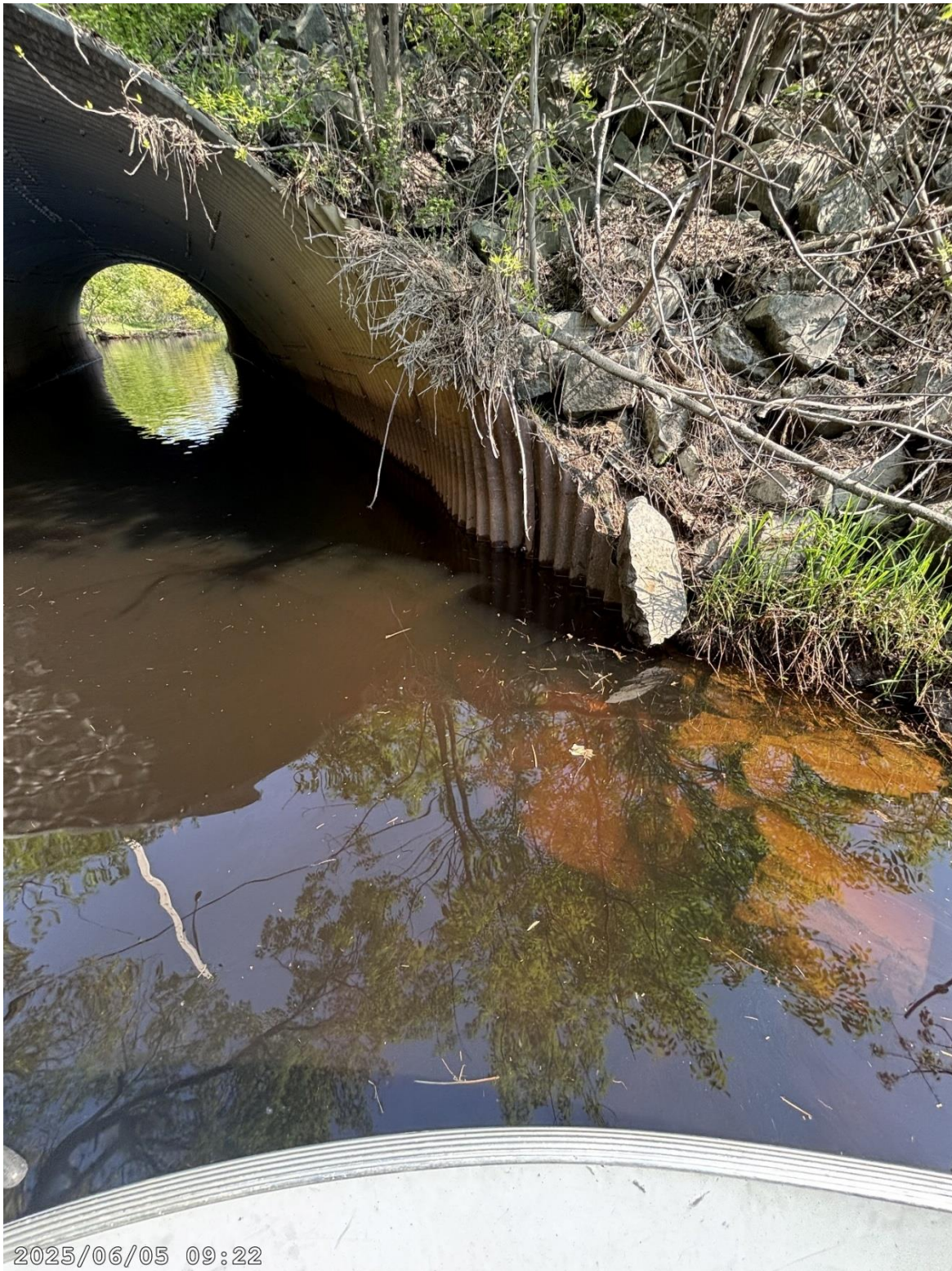
Figure #8: Bulge in Northeast corner of culvert barrel
