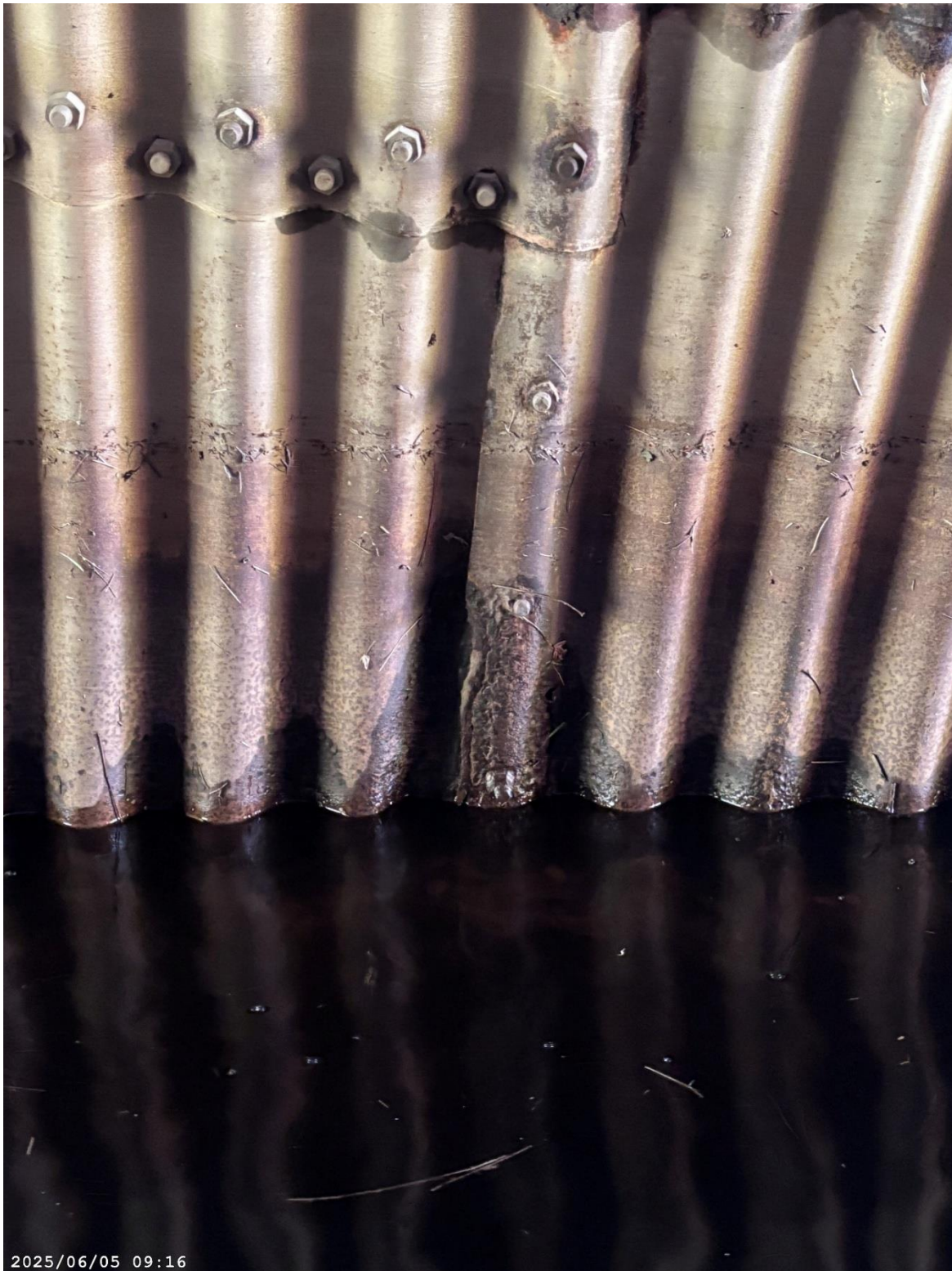
Figure #3: Localized severe flaking of culvert barrel
