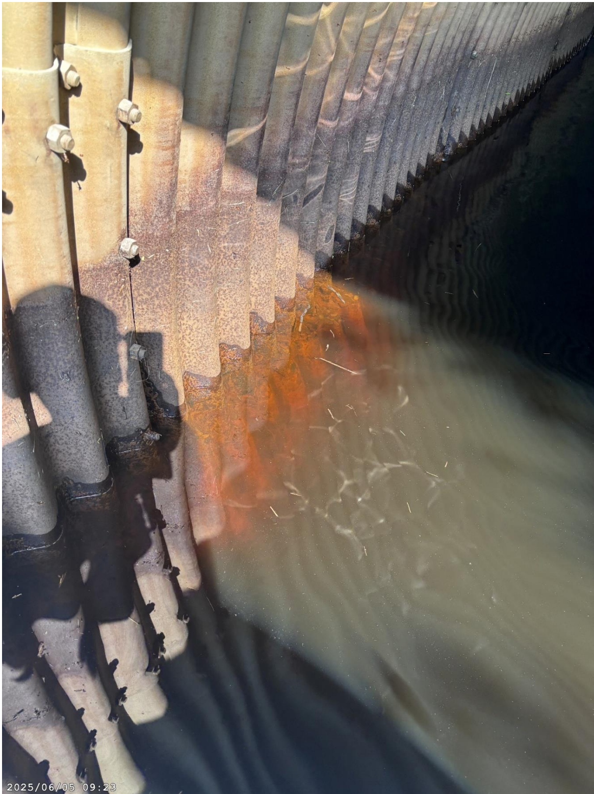
Figure #6: Corrosion of culvert barrel above/below water line
