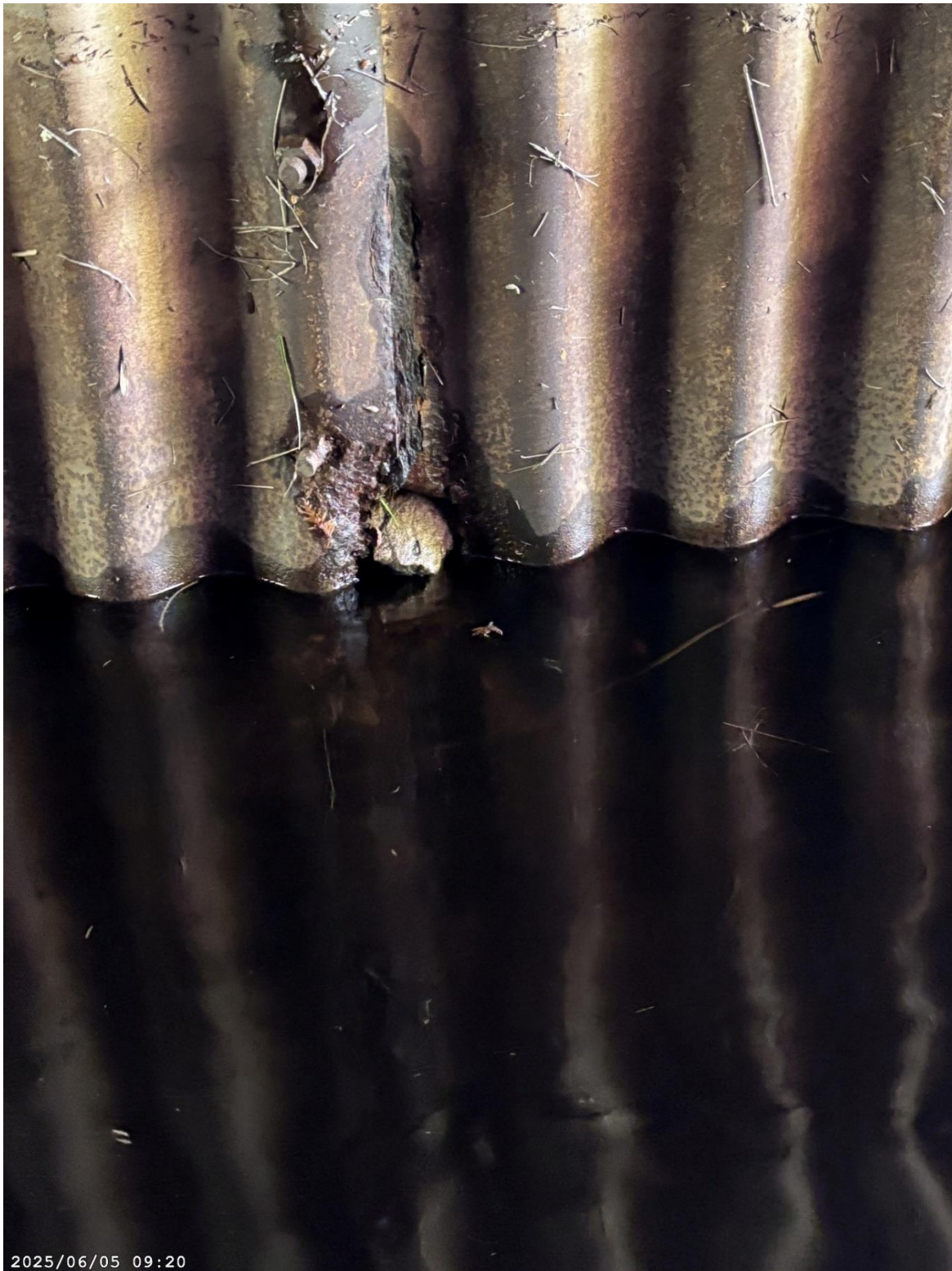
Figure #5: Hole in culvert barrel at water line
